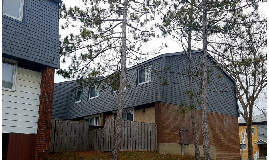
Enviroshingle Installation in Accora Village
