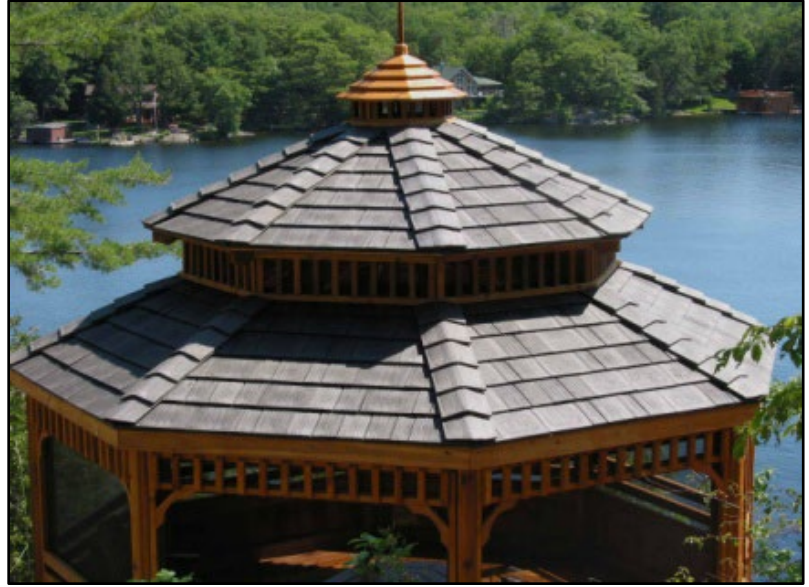
Enviroshake gazebo roof
